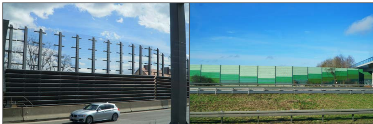
Transparent barriers provide better visual effects to road users and residents.
