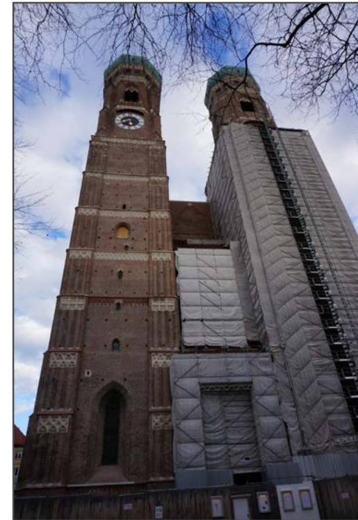
Munich Frauenkirche as a late-Gothic architecture
