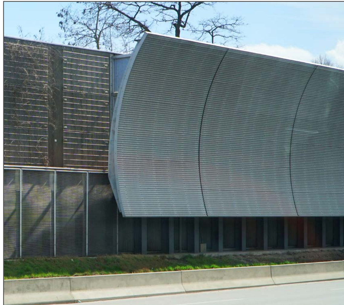
Curved barriers have improved noise reduction while lowered the barrier height.
