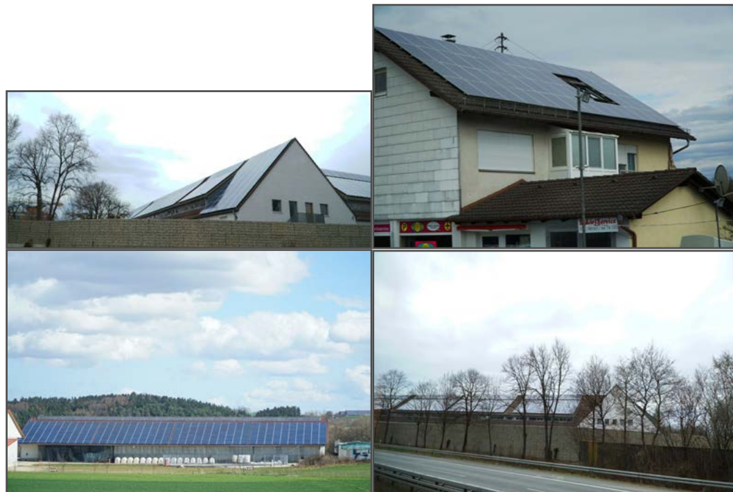
The roofs installed with solar panels, supplying 35% of the momentary electricity demand on sunny weekdays
